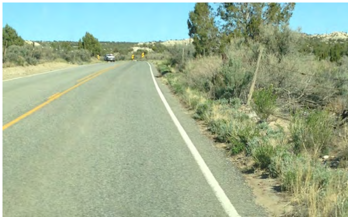
NM 574 – Highway and Right-of-Way Area
