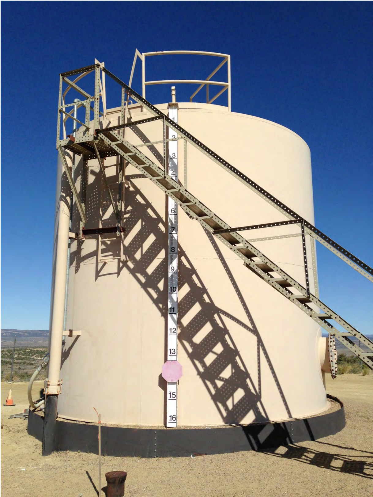
Figure 4: Ground Storage Tank
